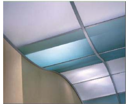
Figure 5.2: Auditorium Ceiling System
